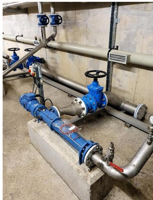
The innovative WANGEN X-LIFT quick-change system ensures reliable pumping of media and a fast rotor/stator change without having to remove any piping. This contributes to a substantial reduction of maintenance costs!
